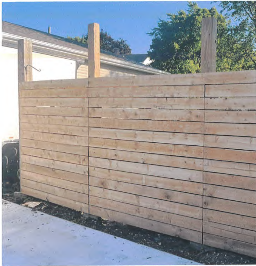
View of exterior fence design (3' x 6" treated panels) looking southeast from 120 Park
